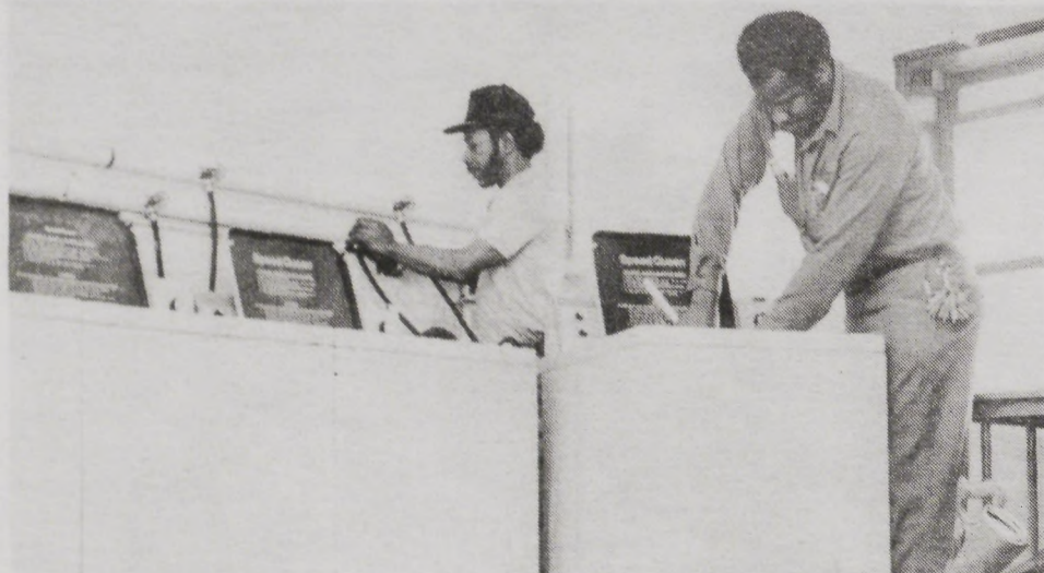
NEW INSTALLATIONS AT NC HOMES. Three new washing machines are being installed by George Williams, superintendent of NC Homes and Palford Drye, Director of Maintenance.
